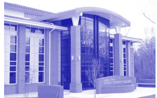
Pictured above: The newly constructed Citizen Services Building, which houses the County's most frequented services.
